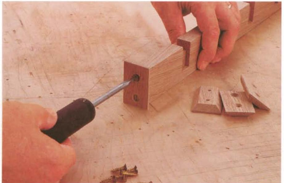
**PHOTO E:** Install the top and bottom end caps with two brass screws.
